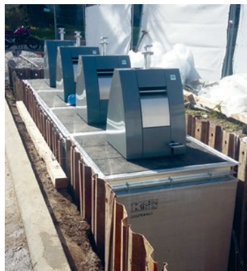
Infrastructure de conteneurs enterrés
